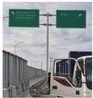
Client : Agung Sedayu Group Location : Pantai Indah Kapuk Service : Road Sign Wayfinding Material : Galvanized Steel, Sticker Reflectif, Pipe 10"
